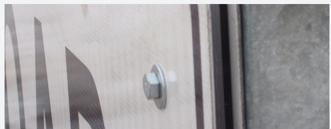
Temporary second sign can be bolted on top of permanent sign.
